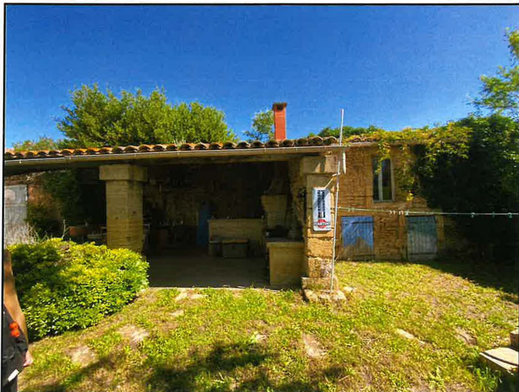
Pool house - atelier - local piscine (23/05/2024)
